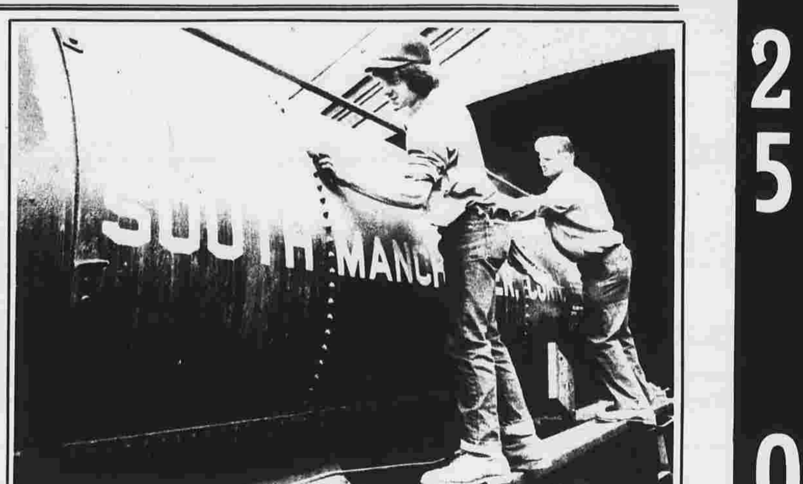
Two workmen raise a cloud of dust as they wipe off what experts say is the last existing car from the old South Manchester Railroad, also known as "Cheney's Goat." The two helped remove the tank car from a brick shed behind the Clocktower Mill building on Wednesday. Both John Hartzell, left, and Max Miller, right, work for the Valley Railroad of Essex - where the car has been donated.
